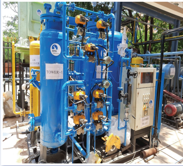
To cater the sudden surge in covid cases during second wave, installed plant for converting “PSA Nitrogen” to “PSA Oxygen” in Gandhi Hospital, Hyderabad, under CSR initiative.
