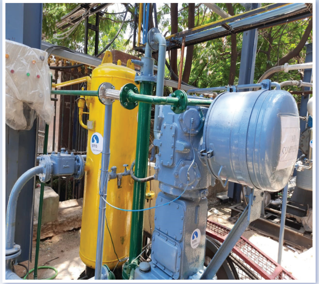
To cater the sudden surge in covid cases during second wave, installed plant for converting “PSA Nitrogen” to “PSA Oxygen” in Gandhi Hospital, Hyderabad, under CSR initiative.
